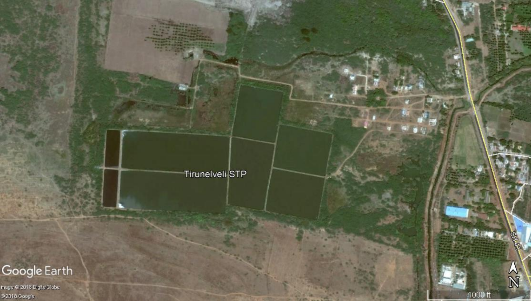
Figure 6: View of Existing Sewage Treatment Plant in Tirunelveli
